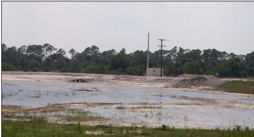
Figure 4. Pump Station S-390 control building, end of discharge pipe and inflow distribution canal (deep zone trench) shortly before construction completion.
