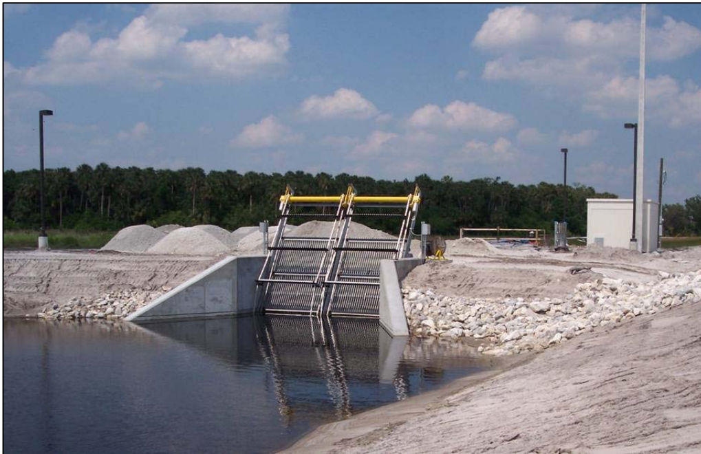
Figure 3. Photograph of S-390 Trash rack and pump station control building shortly before construction completion.
