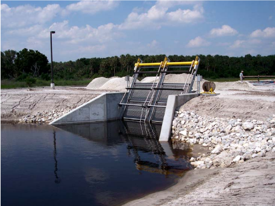
Figure 3. Headwater side of S-390 showing automatic trash rack
