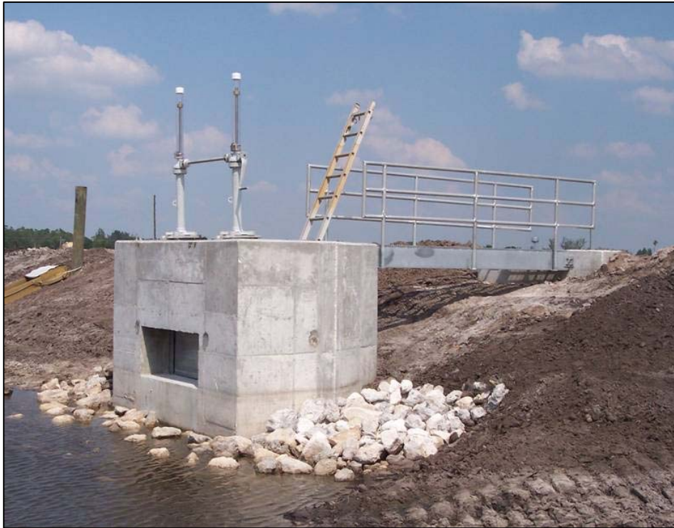
Figure 6. Structure S-391 just prior to construction completion (May 2005).
