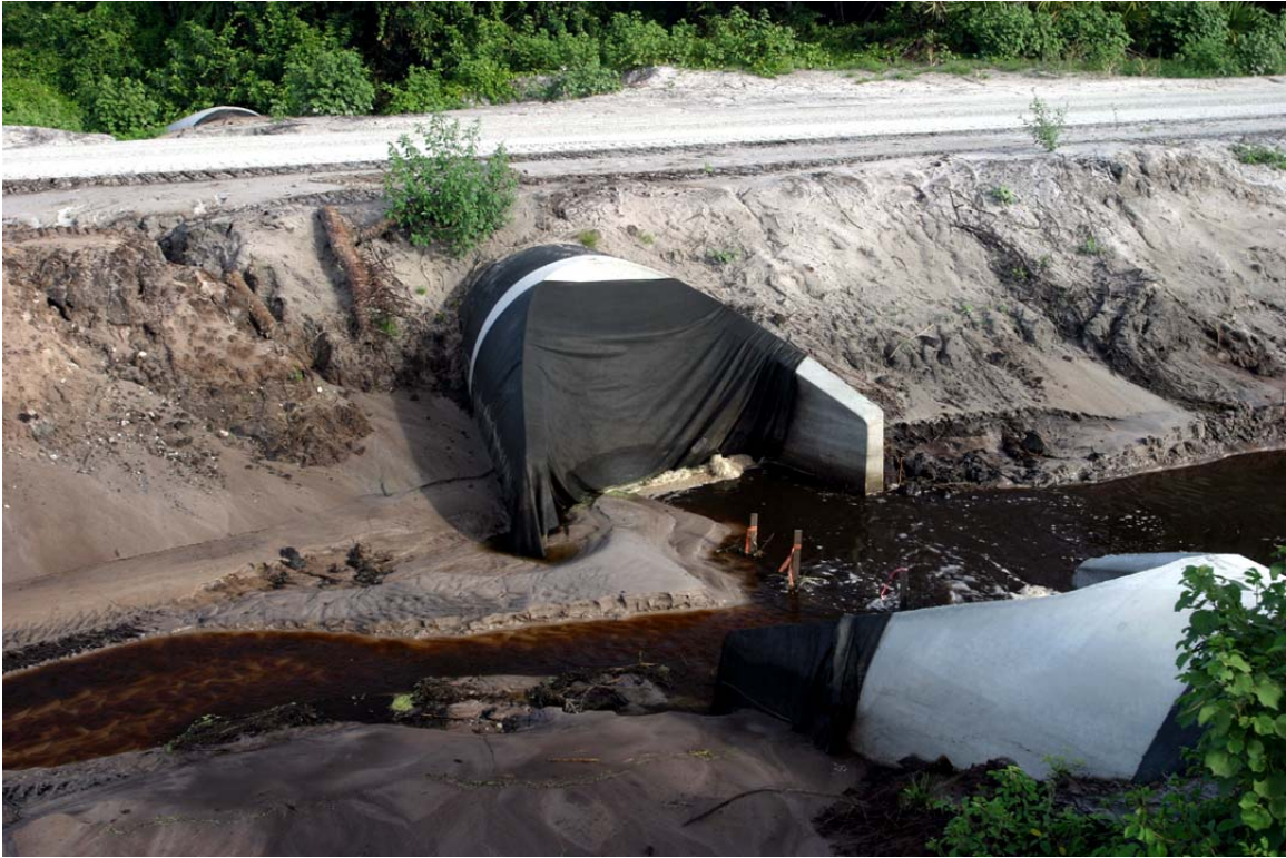
Figure 3. Tailwater side of G-5 structure.
