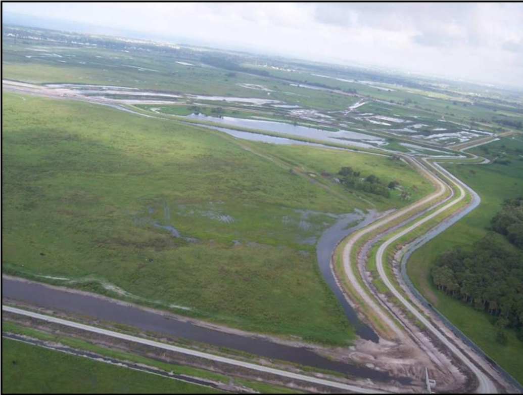
Figure 7. Water enters Cell 1 from the 30-ac storage pond via S-386C, located in the lower right hand corner of the photo. Lake Okeechobee is visible in the background.
