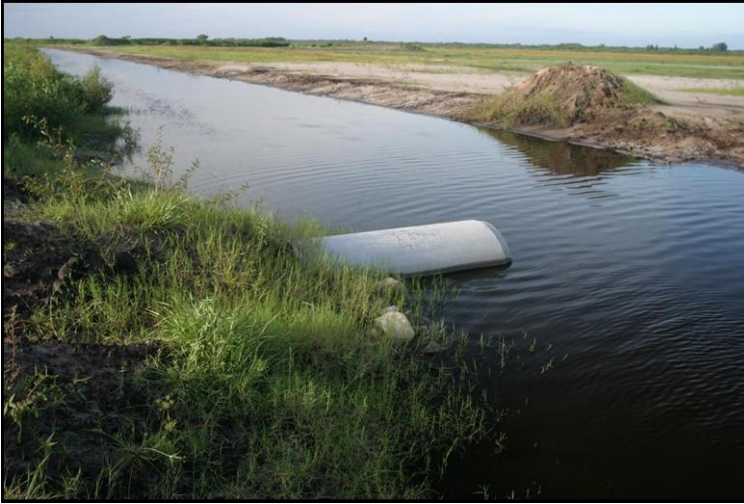
Figure 13. Discharge pipe of S-386B within the distribution canal of Cell 2.
