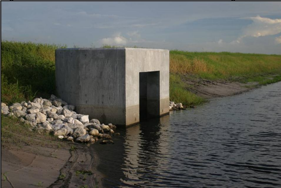
Figure 10. Photo of the headwater side of S-386A during construction.
