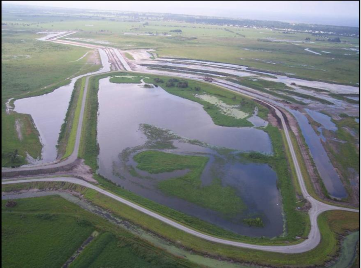
Figure 6. Storage pond looking south. Cell 1 is to the left and Cell 2 is to the right.
