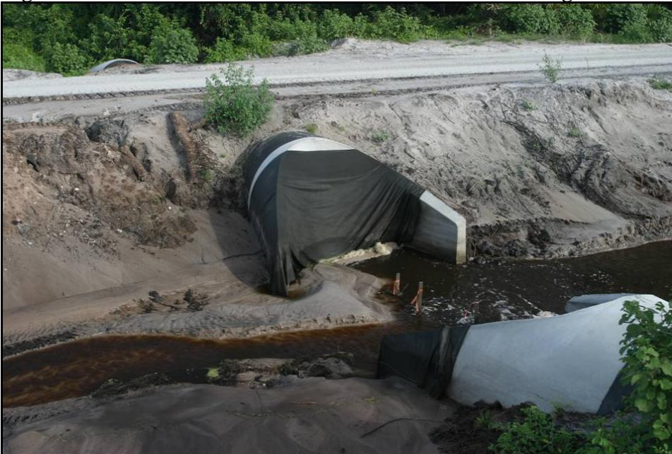
Figure 14. Culvert downstream of Structure S-387B during construction.
