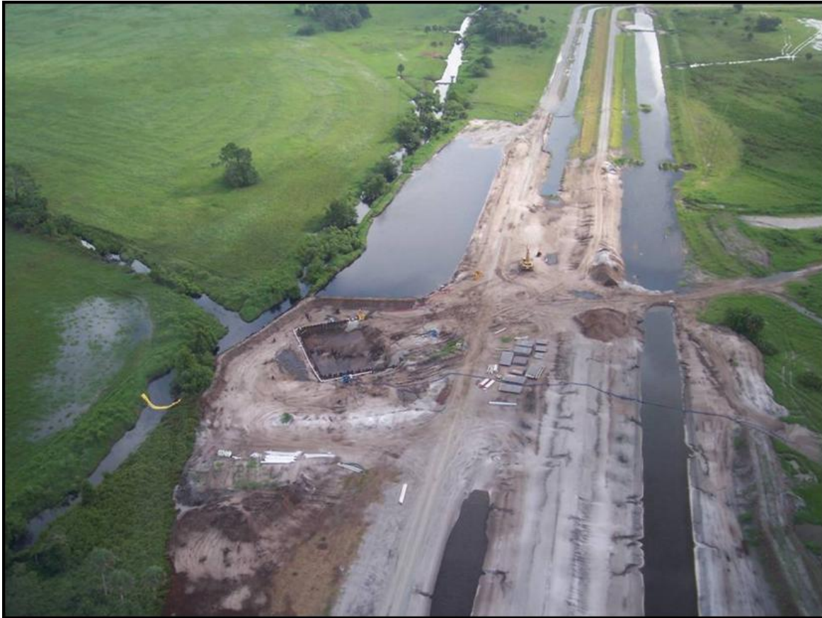
Figure 4. Photograph of S-385 pump station during construction.
